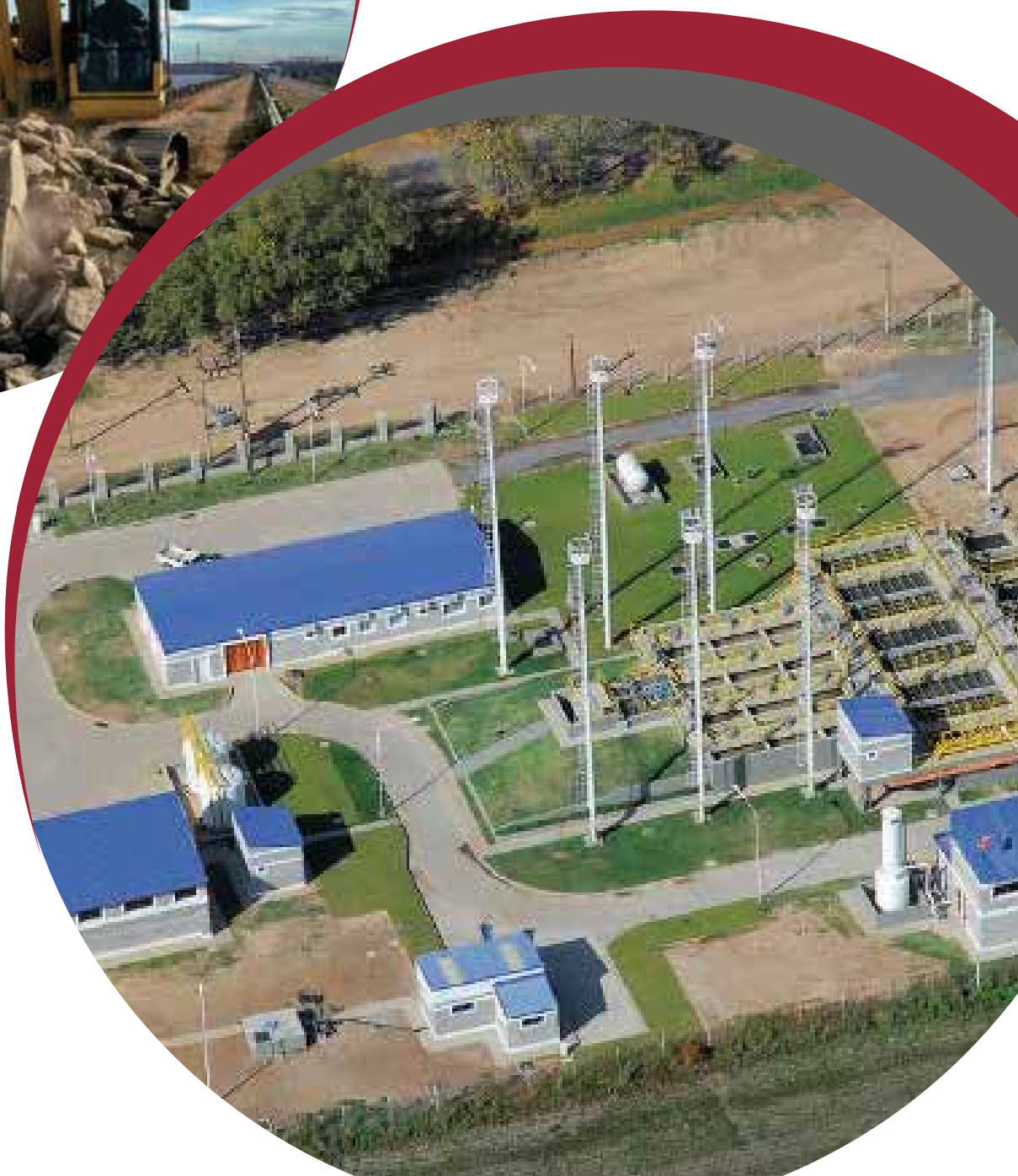
OBRAS DE INFRAESTRUCTURA / INFRASTRUCTURE WORKS
